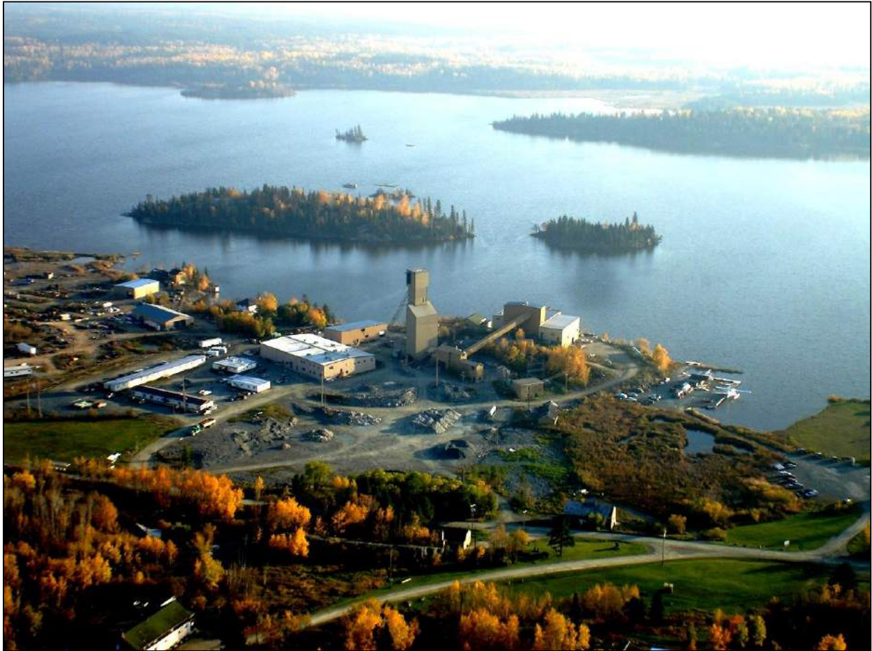
Figure 5.1 Photograph of the True North Gold Mine Looking South
