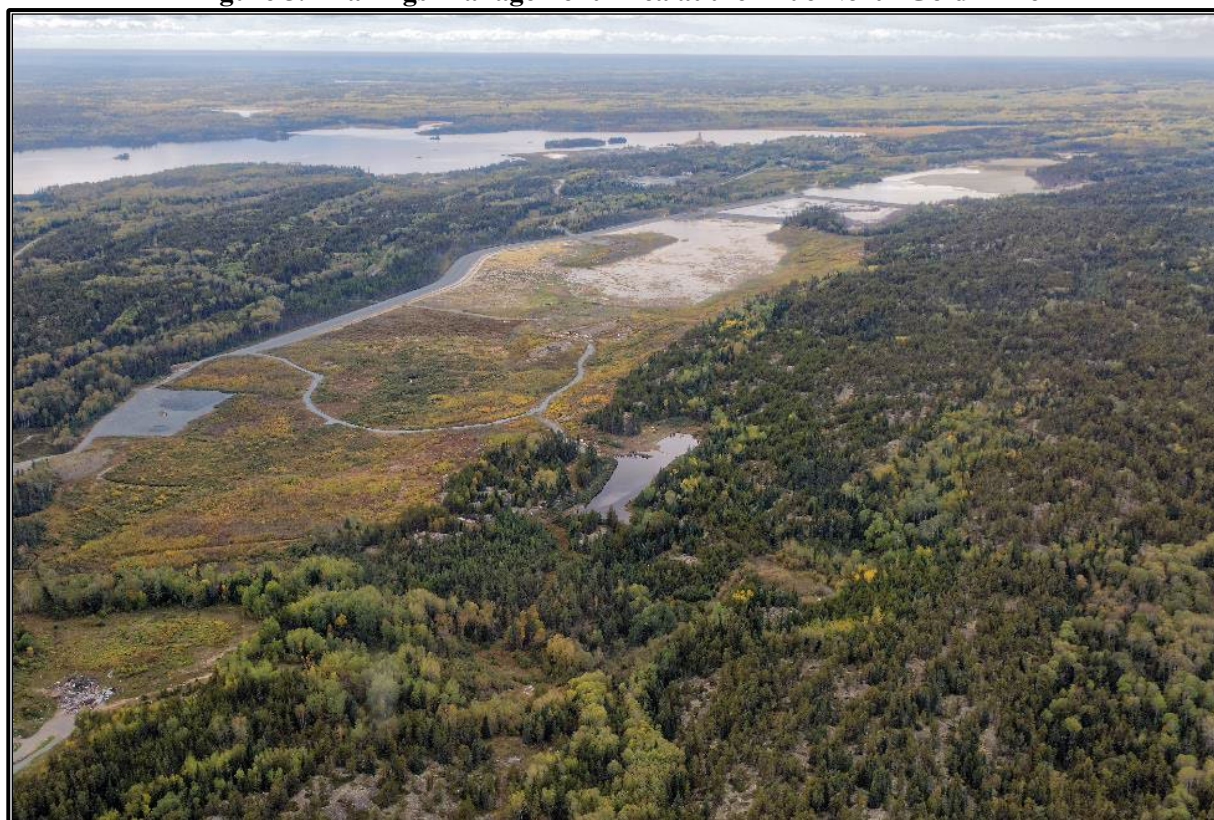
Figure 5.2 Tailings Management Area at the True North Gold Mine
